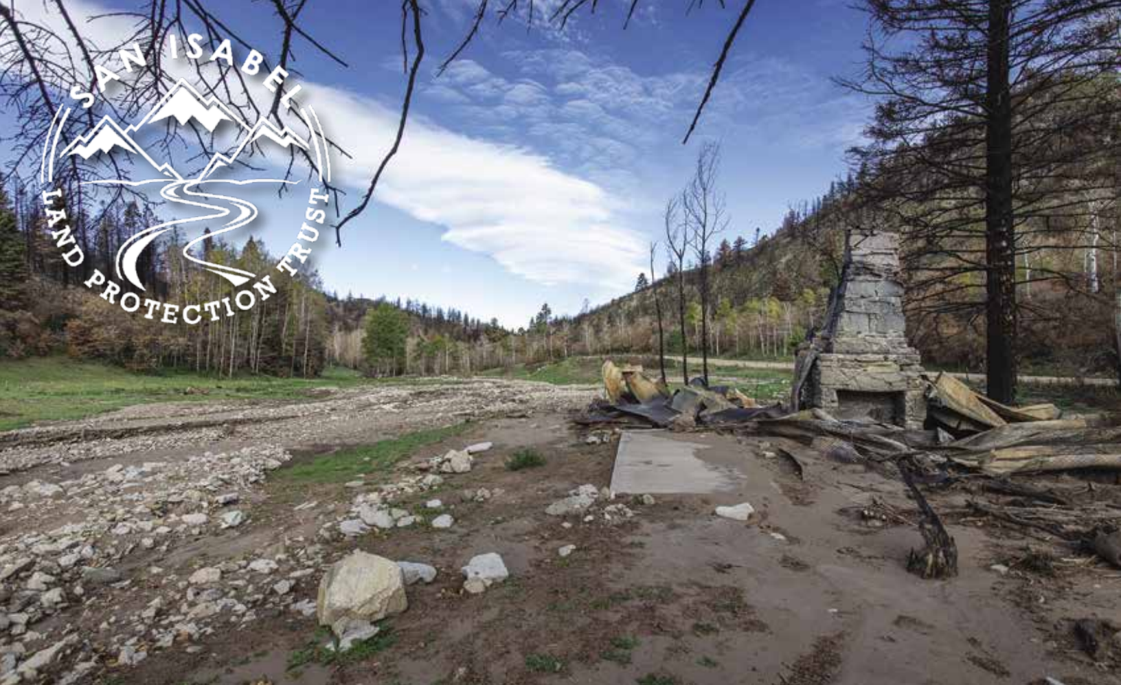
The foundation of a house burned by the Spring Fire sits amid flood and mud-slide debris along Pass Creek Road. (Photos by Greg Smith)
