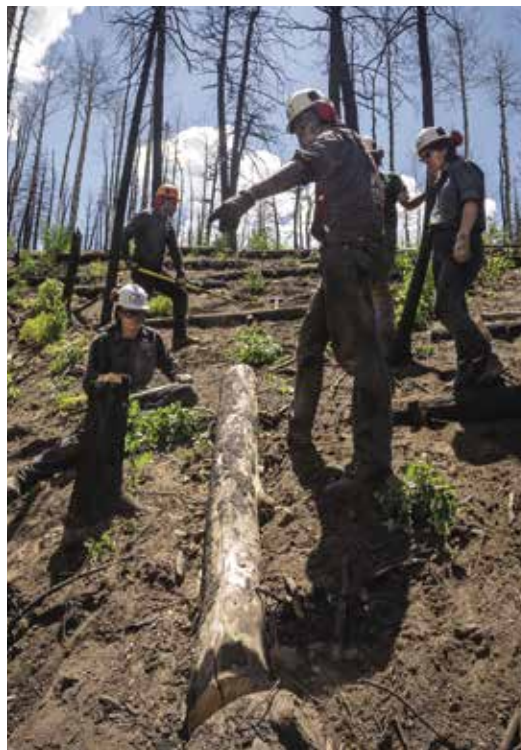
A Mile-High Youth Corps crew stabilizes a hillside on the Thomas property.
